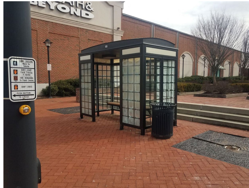
Bus Stop Shelter
